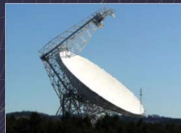
NRAO's GBT the world's largest steerable Radio telescope (105-m in diameter)
